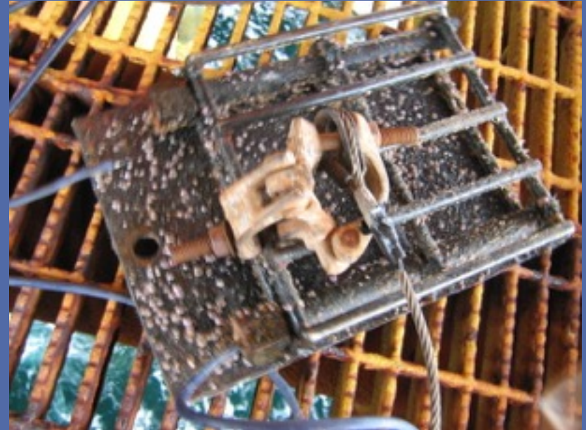
Test Plate – with Activators – power cable broken.
